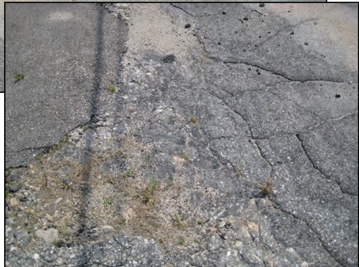
Detail of Poor Pavement Condition
